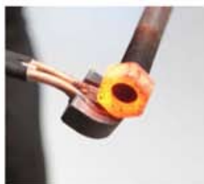
Releasing of rusted bolts
